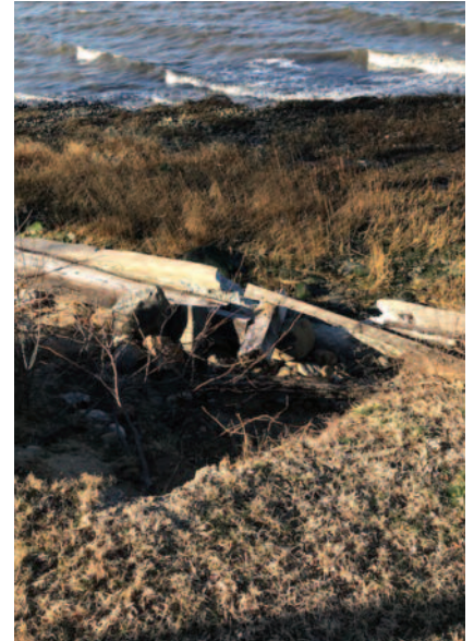
Beneath Arleigh Road
